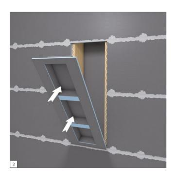
Apply a bead of wedi Joint Sealant onto the exposed stud, as well as along the inside edges of the wall panel.
