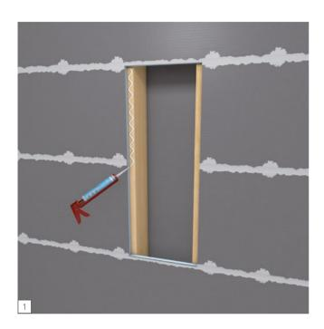
Measure and cut out a space of the existing 10 mm wall panel in an area of 450 mm width so that the Niche Flanges can rest on the framing studs on both sides and line up flush with the surrounding wedi boad.
