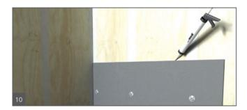
Push the wedi board all the way into the channel of the shower base channel and its bead of sealant. Smooth out any pushed out sealant on inside seam using a putty knife. Fasten the boards directly to the studs starting 300 mm above the base and at a rate of 1 fastener per 300 mm. One extra fastener is set into the seam to the next board to crate a flush transition.
