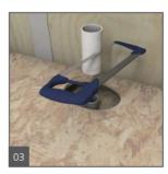
Cut the Adapter 32 mm below the subfloor surface. Make sure that the cut out fits to the Fundo board drain.
