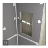
wedi Niches are installed in a cut out in the wedi wall and attached with it's flange right into the center of 16 o.c. studs. wedi sealant is set along the connection of wall to niche.
