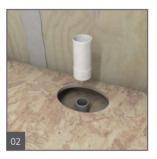
... to allow wedi drain trap to be inserted and connected to floor pipe using appropriate ABS compatible or multipurpose cement glue. Please also check cement glue compatibility to floor pipe material. The drain and trap have to be secured to the subfloor. Drain recess cut out must not add deflection to subfloor.
