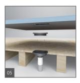
Glue and seal the wedi drain trap to the DN 50 pipe. Mount the sealing collar to the wedi Riolito neo underside counterpart using a manual phillips screwdriver.
