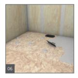
Apply a skim coat and finally a combed through bed of a thinset using modified thinset and a  $10 \times 10$  mm notch trowel.
