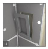
2 Fasteners each side of the niche are set to create a flush transition to the wall boards. Another 10 mm bead of wedi sealant is spread over fasteners and seams.
