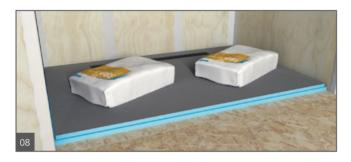
Press the Fundo firmly into the thinset bed, ensuring that the installation is level and void free. Ensure wedi drain's sealing gasket is firmly inserted in the wedi trap with no chance that thinset could have pushed into this connection area.
