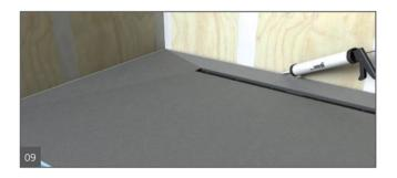
Set up a continuous 10 mm bead of wedi 610 adhesive sealant at the perimeter channel and only in areas where you can immediately install a wedi Building Board into the fresh sealant.
