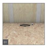
Cut DN 50 pipe minimum 70 mm below the top of the Subfloor. Use the oval shape cutting template to cut subfloor using a jigsaw. Position the oval template according to the position of the Riolito model's predetermined position f its drain location, relative to the squared wall framing...
