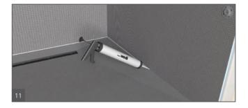
Apply continuous 10 mm beads of sealant between all connections of boards and install with tightly butted seams. Excess sealant must be spread flat with a putty knife. All seams and fastener heads in the assembly are covered with a secondary 10 mm bead of sealant and spread flat. The seams should be covered to 25 mm on either side of seam. All fastener/washers are covered with sealant stretching 25 mm over the washer edges.
